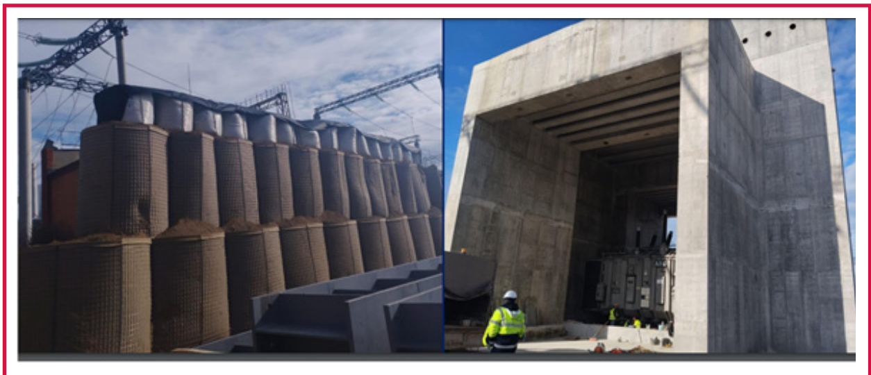
Examples of engineering protection of the 1st (left) and 2nd (right) levels of CEI facilities.
