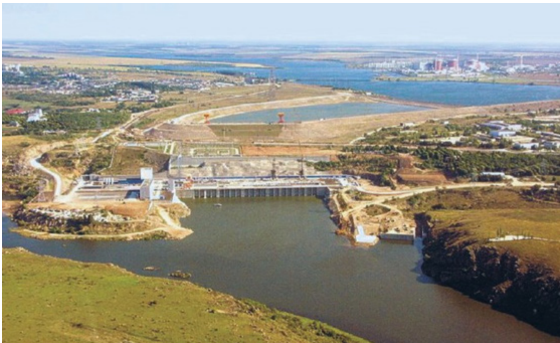
Panorama of the Tashlyk pumped hydro storage power plant, which forms an energy complex with the South-Ukrainian NPP
