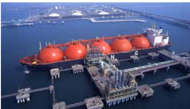
Fig.3. Gas liquefaction plant in Damietta
