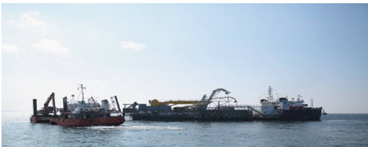
Photo 1. The working process of the cable laying vessel and auxiliary ships OSK-ShipTech in the Baltic Sea
