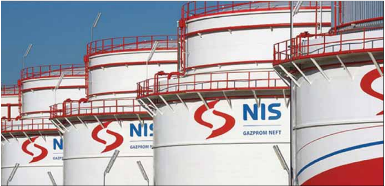
Photo 1. NIS (Gazpromneft affiliate) tanks Source : https://www.gazprom-neft.com
